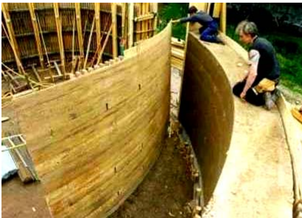
Construction of the Chapel of Reconciliation, Berlin 2000 Earth Builder Martin Rauch Πηγή: University of Research Sydney, Earth Building Research Forum
